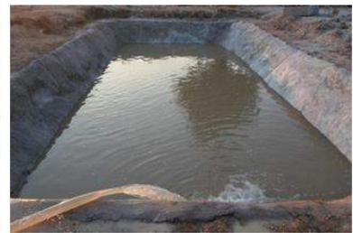
A comparison of the expenses for building the two pools with 10 meters long, 5 meters wide and 2.5 meters deep (trapezoid) was made and showed that the cost of a concrete pool is higher than a soil cement pool at 38% because the concrete pool is reinforced iron and wall, making its floor thicker than the soil cement pool while the soil cement pool is in contrast coated with soil cement along the wall and floor, for the soil cement cannot be casted like concrete.
